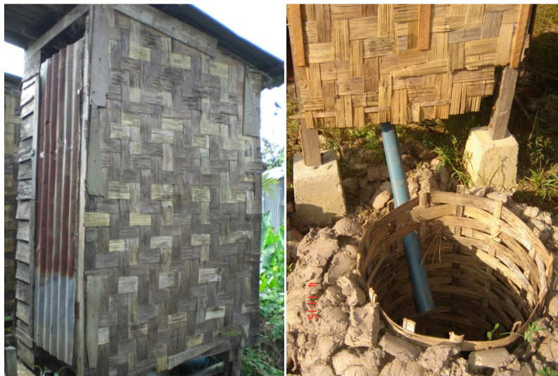
Figure 5: (LHS) A typical pit latrine in villages in Yangon. The pit latrine is constructed of bamboo sheets and thin planks of wood. (RHS) Each pit is typically eight feet in depth with a woven bamboo basket in place for wastes.
