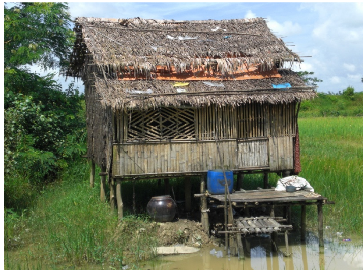
Figure 2: A typical house in villages in Yangon. The houses are usually constructed of bamboo sheets and thin planks of wood. Earthen vats in front of the houses are used to store water collected from ponds.
