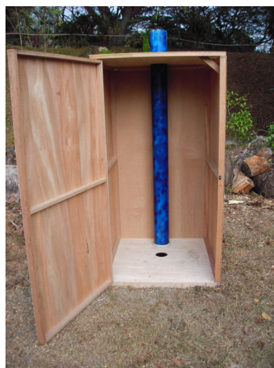
Figure 7: A full-scale pit latrine in SRCS campsite.
