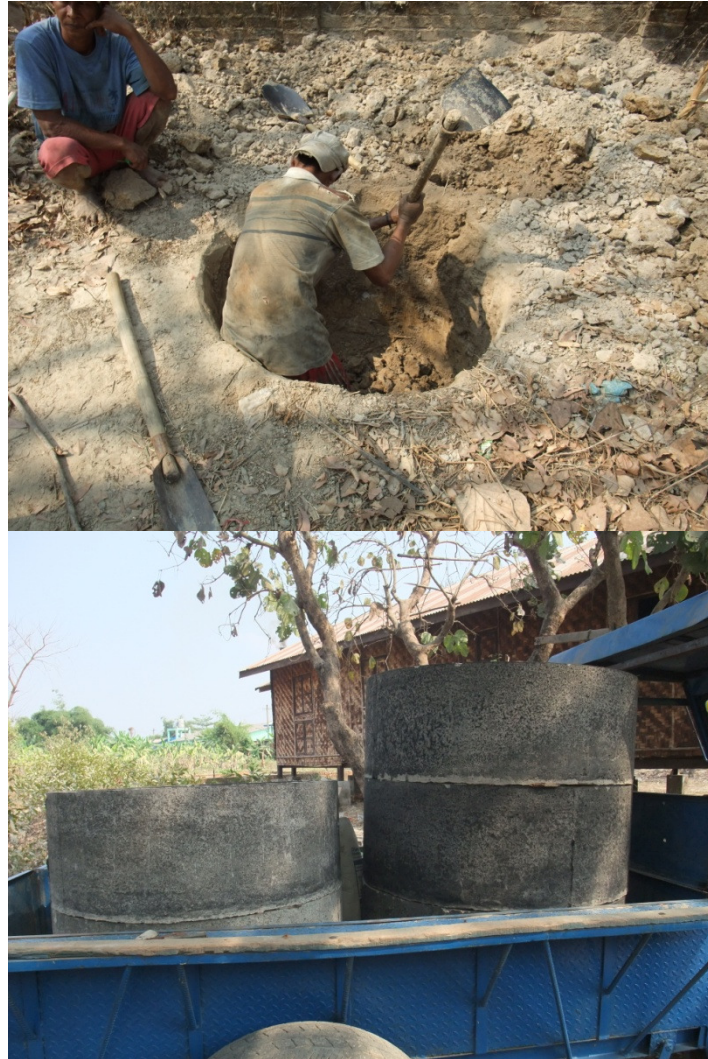
Figure 8: (Top) A Myanmar worker digging the pit for the sanitation system. (Bottom) Concrete rings that will be placed in the pit to contain wastes from the latrine. The concrete rings will minimise risks of contamination of nearby water sources like ponds.
